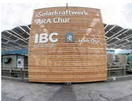
Facade of the solar roof. Image: dhp technology
